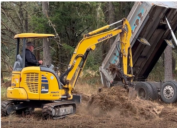
Breaking ground at the McMahon Home Build, October 2022
